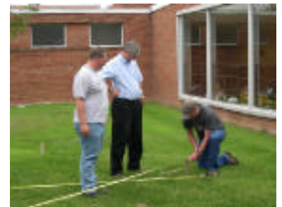
Curt Swineford and Bart Gill conduct surveying work at the high school, while Richard Stump, retired agricultural educator and Center field representative, supervises their work.
